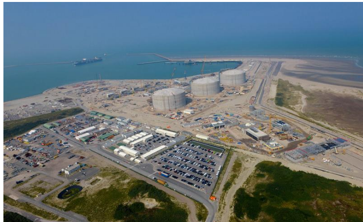
Figure 18: Work site of the methane tanker terminal and Clipon beach
